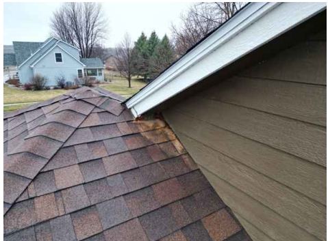
Southeast Above Garage
