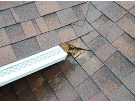
East above garage
