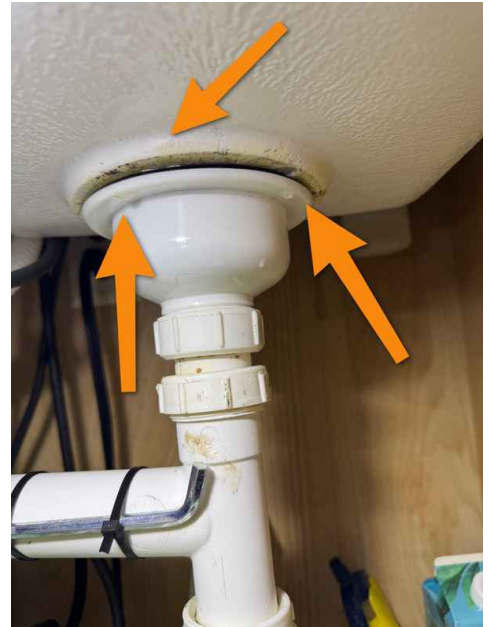
1st Floor Kitchen
